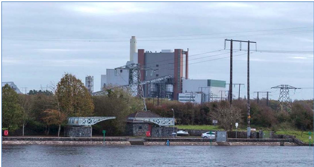
Figure 14-13 View of the West Offaly Power station from across the Shannon
